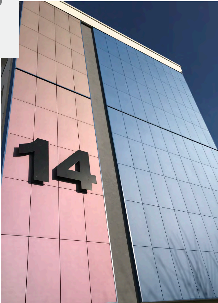
Port 9 Apartments (FR) # Architect: studio A3 # Aquila MATT, colour Iridescent Lilac (9932) & Turquin (5017)
