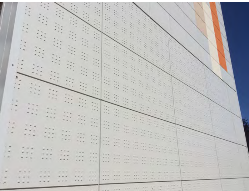
Le Moulin Liot Apartments (FR) # Architect: Boucheron Architecture JBA # Aquila CARVI & Alpha PIERRE DE LOIRE, colour Silver (90)
